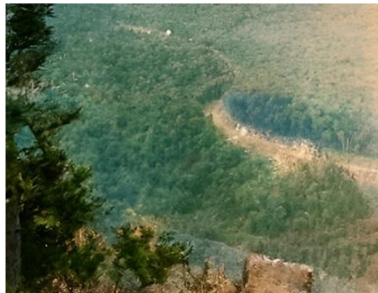
1928 view west at lowered alignment under construction - AMC Archive
